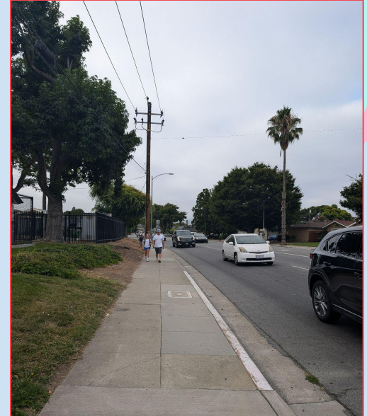
Narrow sidewalks (with obstruction ) on Leigh Ave.
